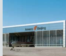
Ameco A380 Hangar Peking, China
